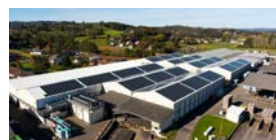
Centre PV Cooplim
